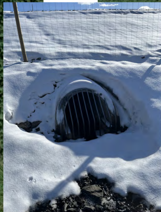
Trumma under JV B: 800mm H: 1000mm
