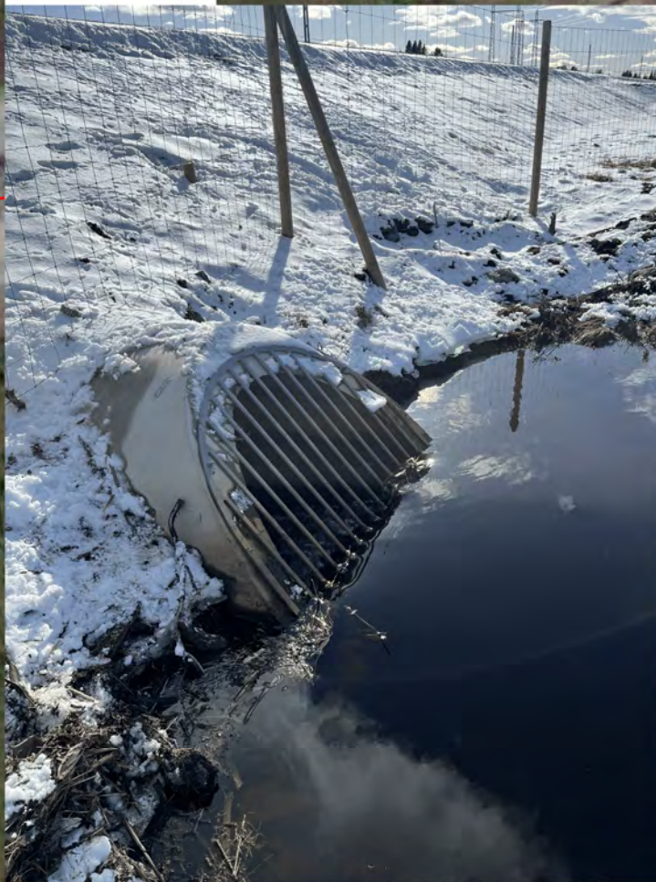
Trumma under JV B: 1400mm H: 1400mm
