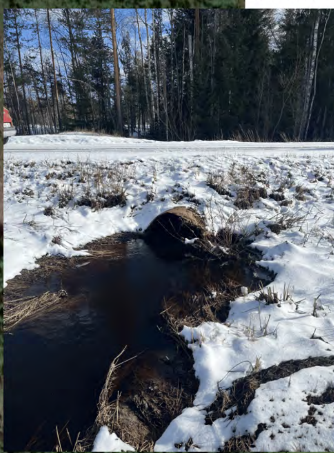
Trumma under GC D: 1000mm
