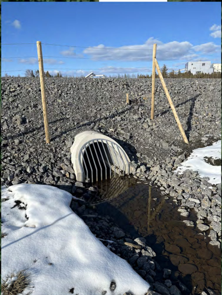
Trumma under JV B: 800mm H: 1000mm
