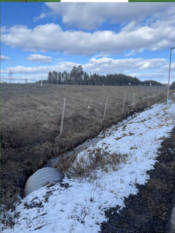
Trumma under GC D: 1000mm
